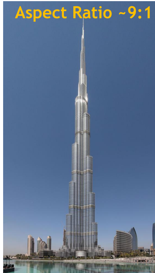
The Burj Khalifa, tallest structure in the world
